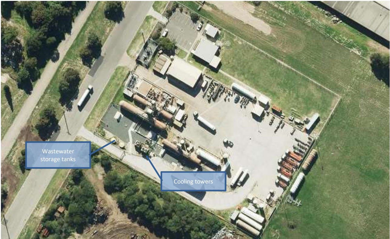
Figure 3-2: Location of BOC Kooragang’s cooling towers and wastewater tanks
