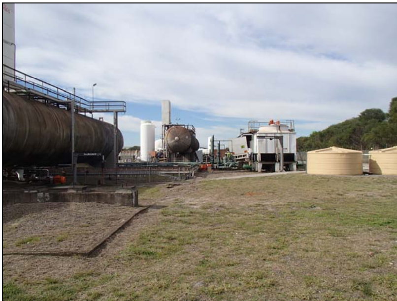
Figure 2: View looking east from CPT 302 to CPT 301
