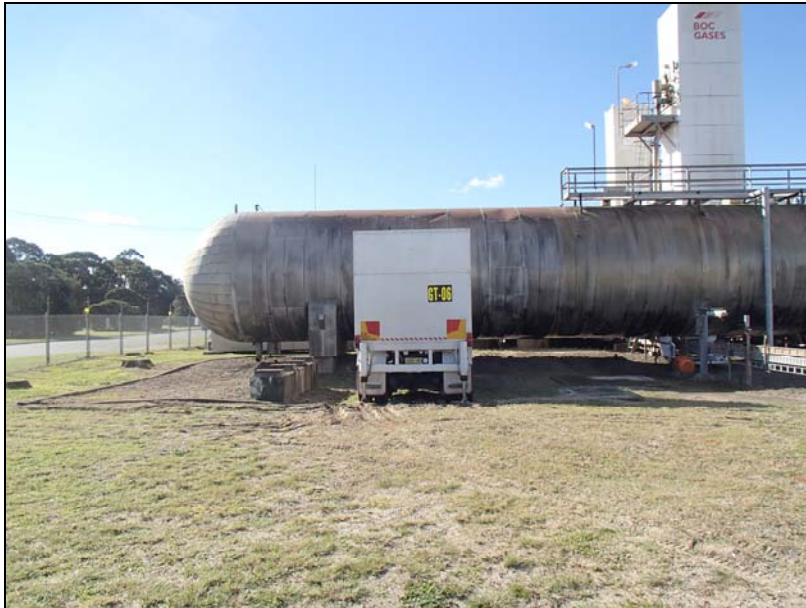
Figure 1: View of site at CPT 302
