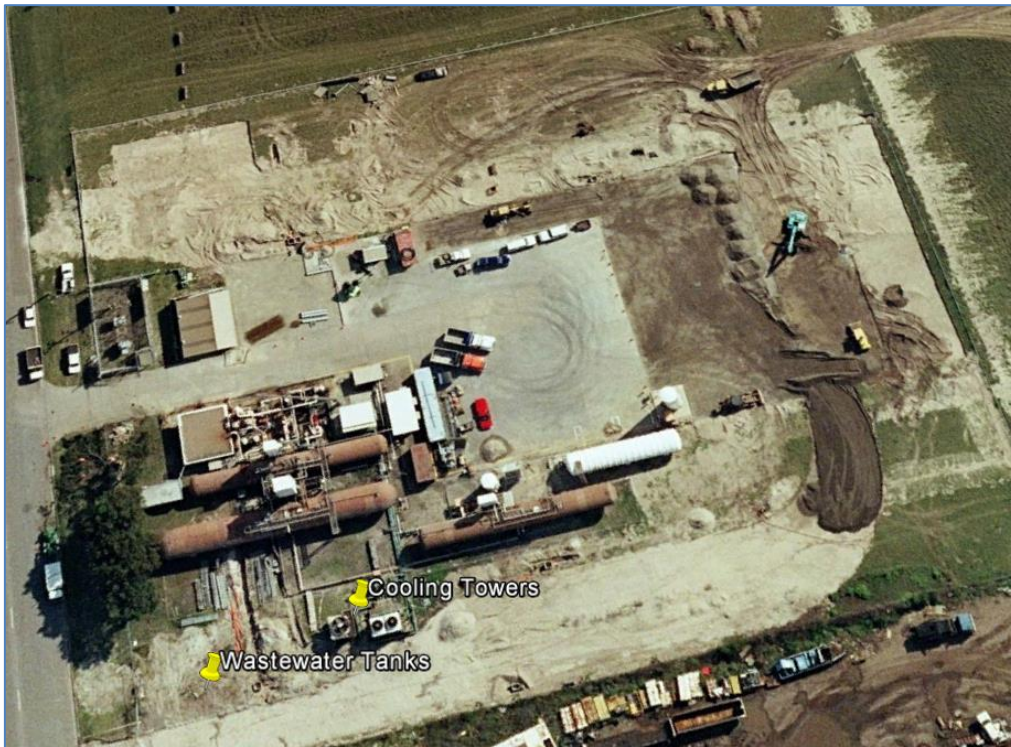
Figure 2-2: Location of BOC Limited’s Cooling Towers and Wastewater Tanks
