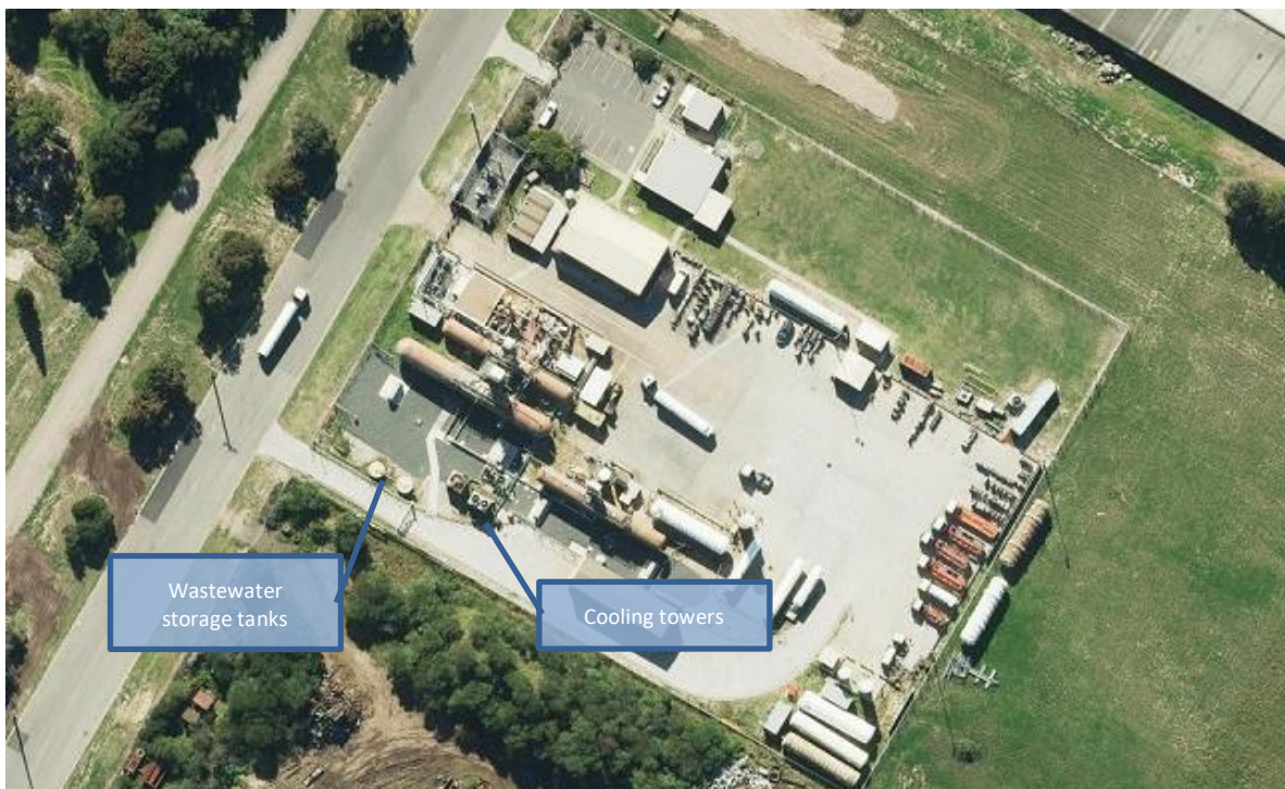
Figure 2-3: Location of BOC Kooragang's cooling towers and wastewater tanks
