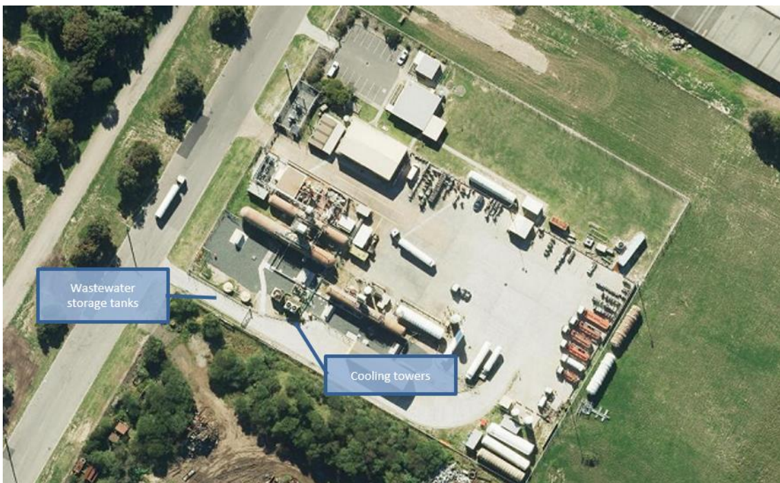
Figure 2-2: Location of BOC Limited's cooling towers and wastewater tanks
